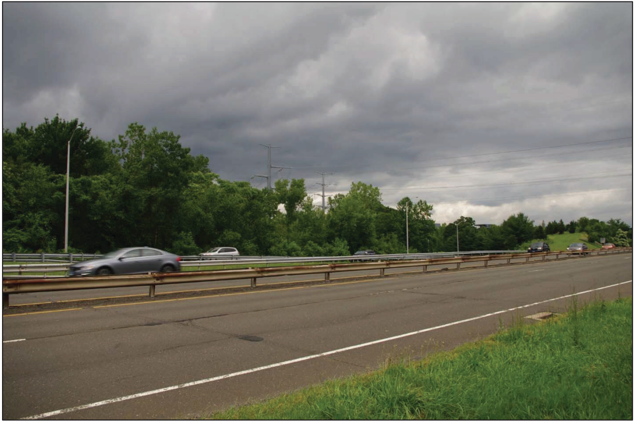
Photograph 2: Merritt Parkway between Perry Avenue and the Route 7 interchange, camera facing northeast.
