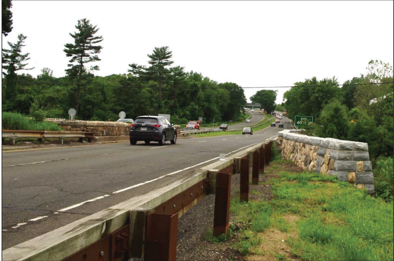
Photograph 7: Merritt Parkway Main Avenue Bridge (Bridge Nos. 530A and 530B), Parkway level, camera facing west.
