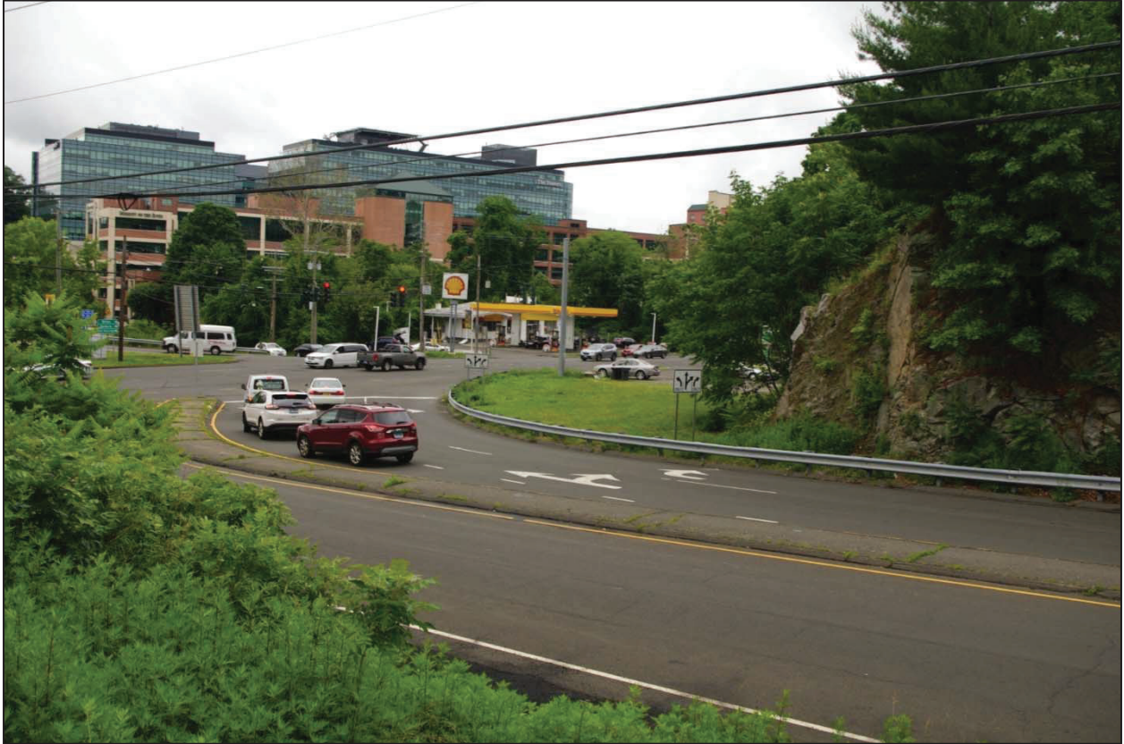
Photograph 4: Merritt Parkway on ramp and off ramp at the interchange with Main Avenue, looking northwest toward the intersection of Main Avenue and Glover Avenue.
