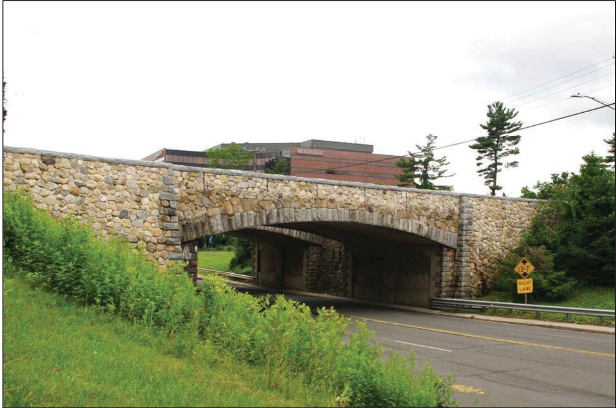
Photograph 5: Merritt Parkway Main Avenue Bridge (Bridge Nos. 530A and 530B), north elevation, camera facing southwest.
