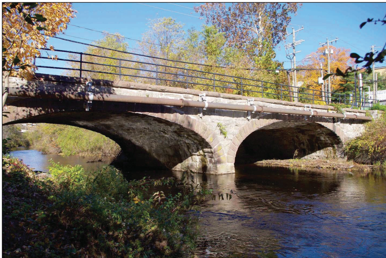
Photograph 10: Glover Avenue Bridge (Bridge No. 004155), south elevation, camera facing northeast. This bridge, which would be replaced under both build alternatives, is evaluated in a separate 4(f) document using the Nationwide Programmatic Section 4(f) Evaluation and Approval for FHWA Projects that Necessitate the Use of Historic Bridges.
