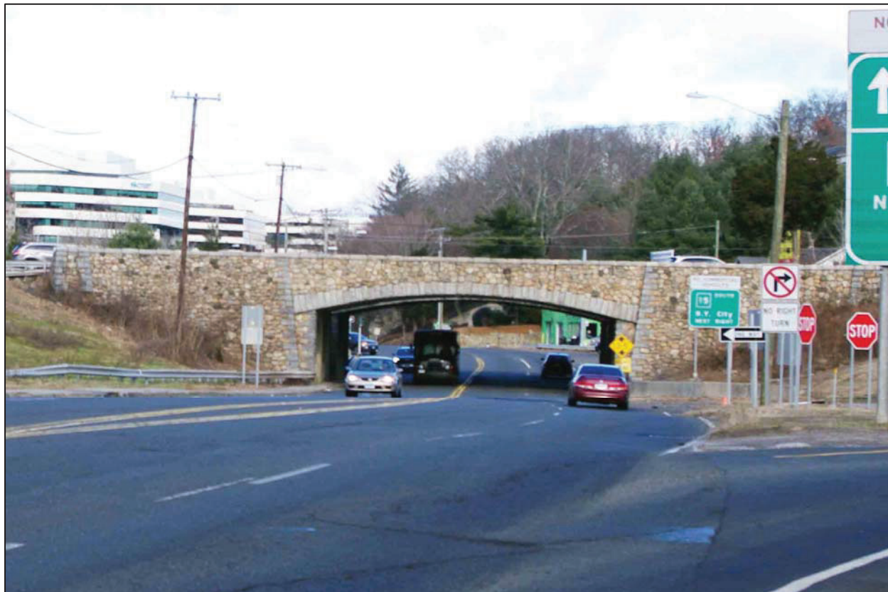
Photograph 6: Merritt Parkway Main Avenue Bridge (Bridge Nos. 530A and 530B), south elevation, camera facing north.
