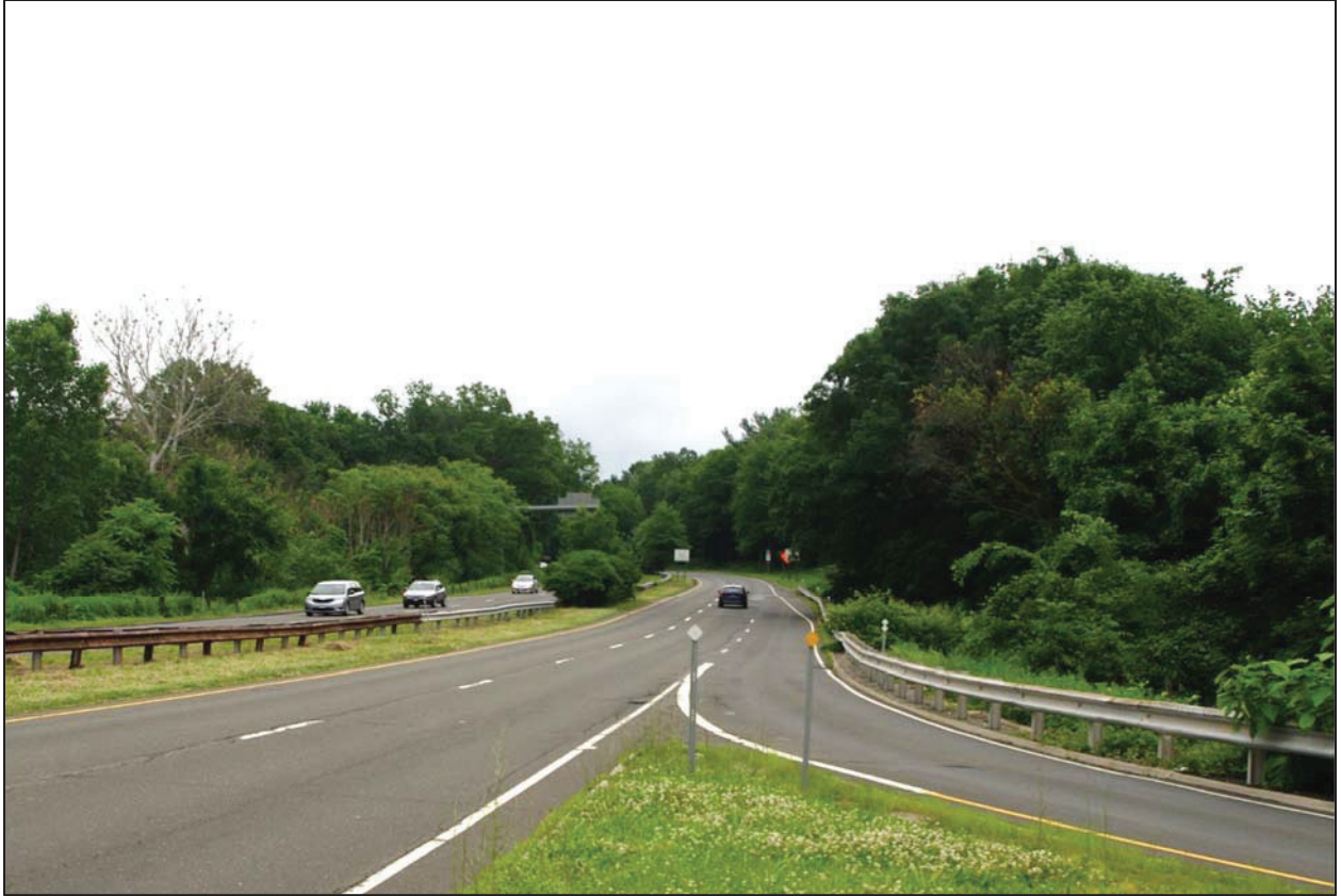
Photograph 1: Merritt Parkway north of the Main Avenue interchange, camera facing northeast.
