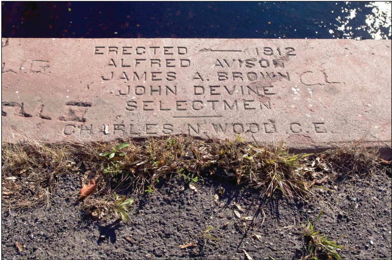
Photograph 11: Dedicatory inscription, Glover Avenue Bridge, south parapet. The project's MOA calls for the re-use of this stone in the new bridge.
