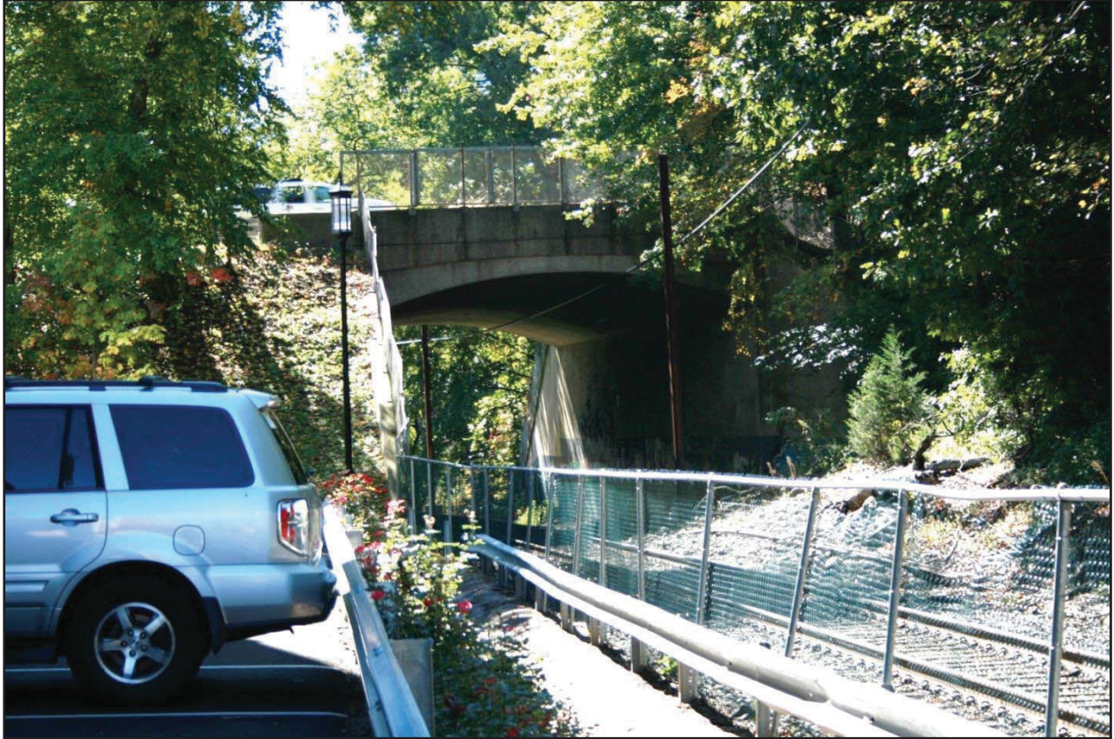
Photograph 8: Merritt Parkway Metro-North Bridge (Bridge No. 720), north elevation, camera facing south.
