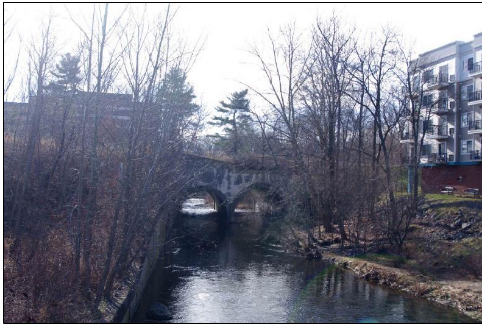
North side seen from Glover Ave bridge, facing south. This view would be obscured by a ramp
