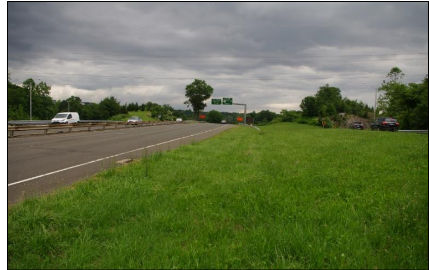
East of Perry Ave undergrade bridge, facing northeast. The Parkway-to-Route 7 Southbound ramp is at the right. Signs for upcoming exits are in the distance
