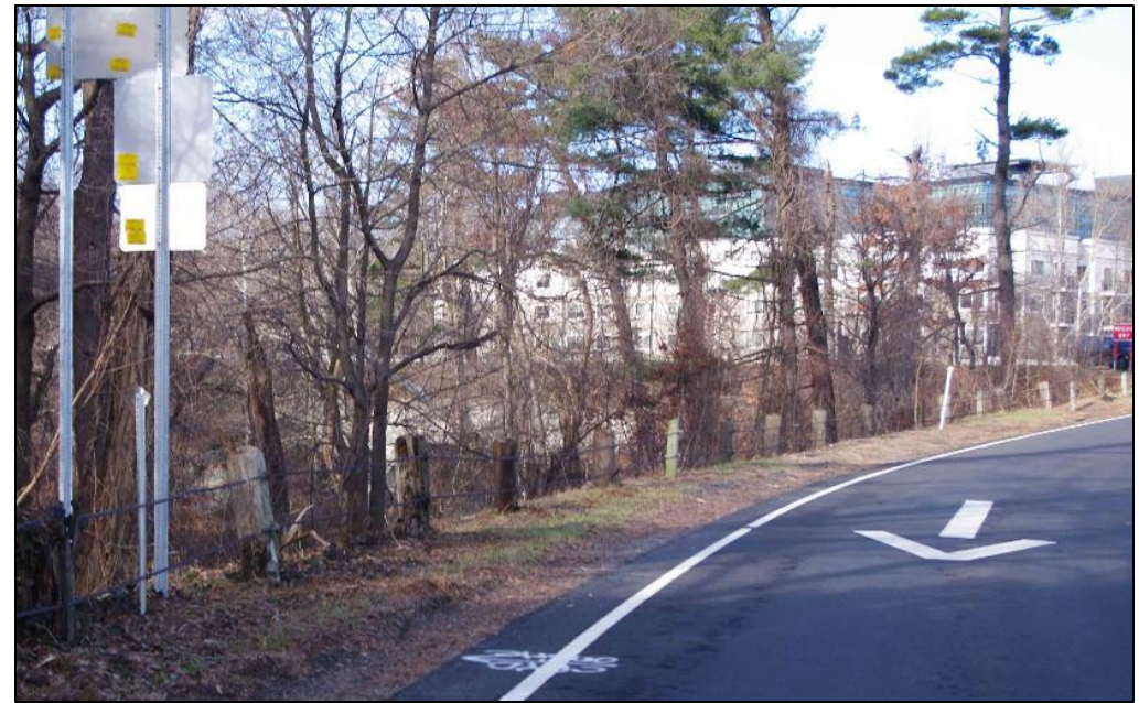
South side, from parkway exit ramp, facing northwest
