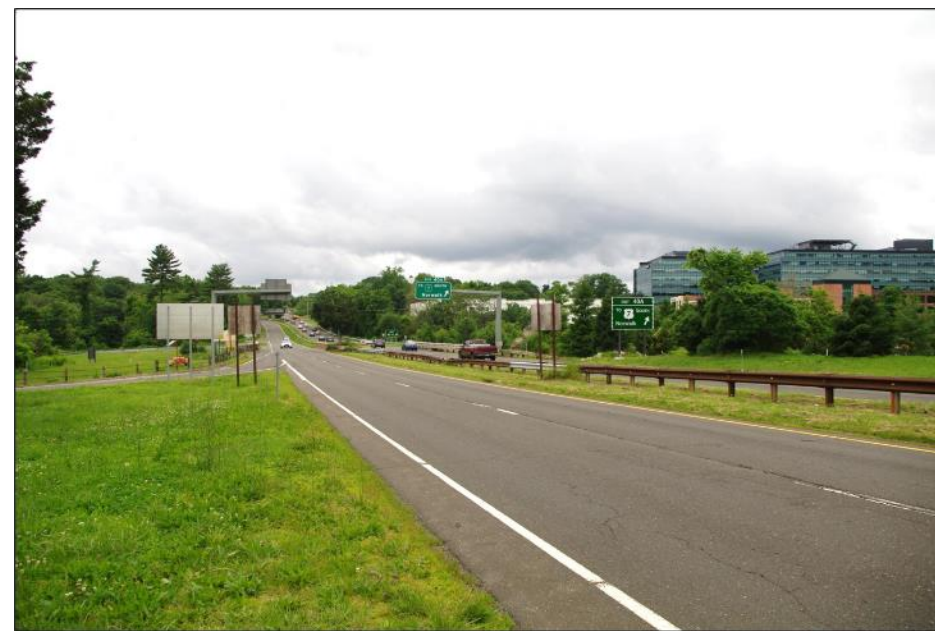
Parkway north of the Main Ave interchange, facing west
