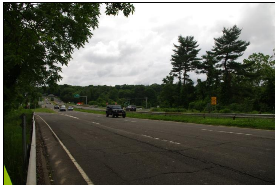
Character of the Parkway between the ramps for Route 7 and the ramps for Main Ave, facing east
