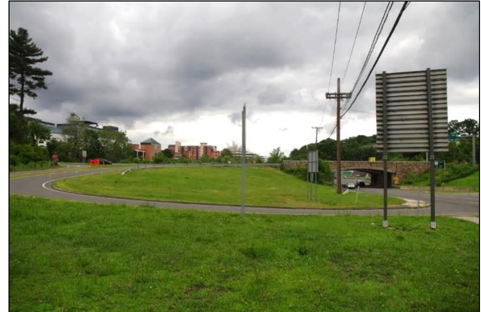
Overview of the on-ramp in the southwest quadrant, facing north, south elevation of the Main Ave bridge at right
