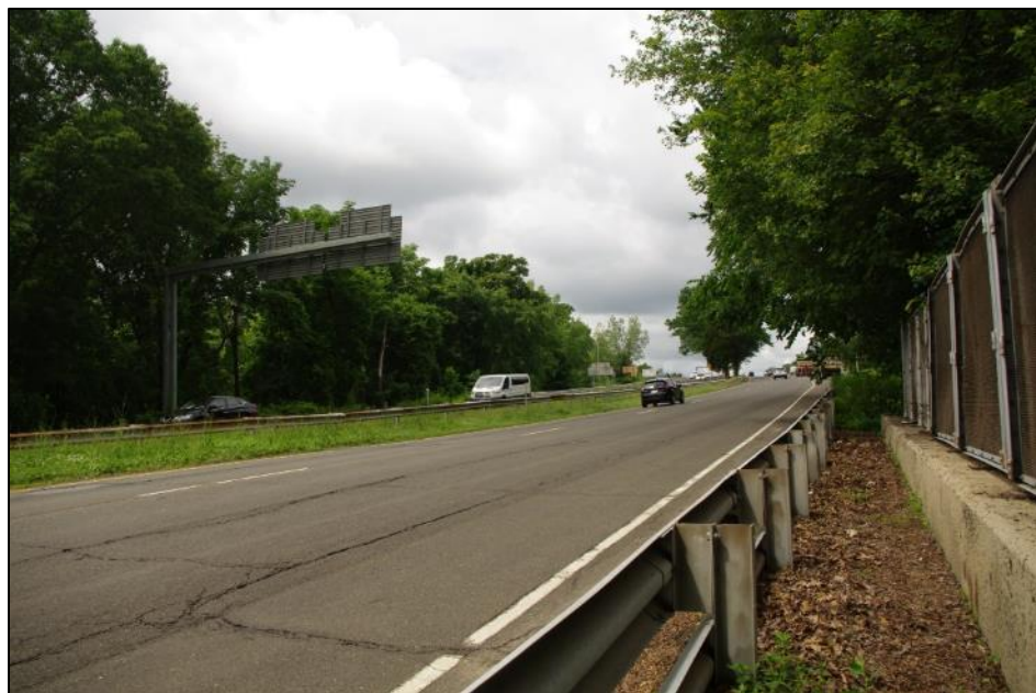
Parkway between the ramps for Route 7 and the ramps for Main Ave, facing southwest. The concrete parapet with metal screening is the Metro-North bridge
