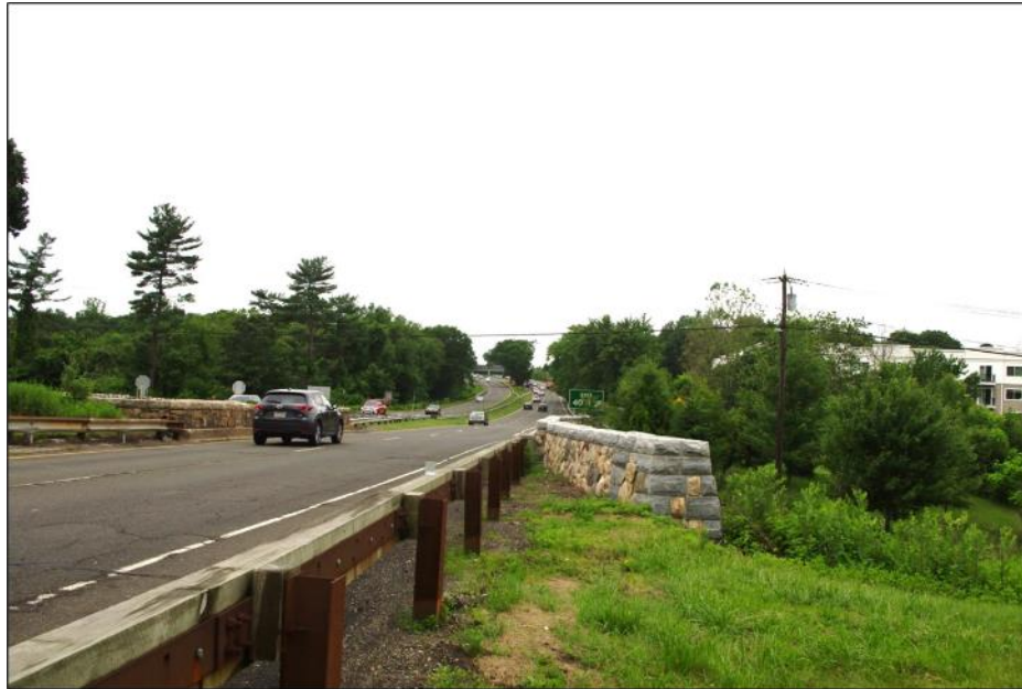
Detail of the timber-on-metal guiderail, joining up with the parapets of the Main Ave bridge, facing southwest
