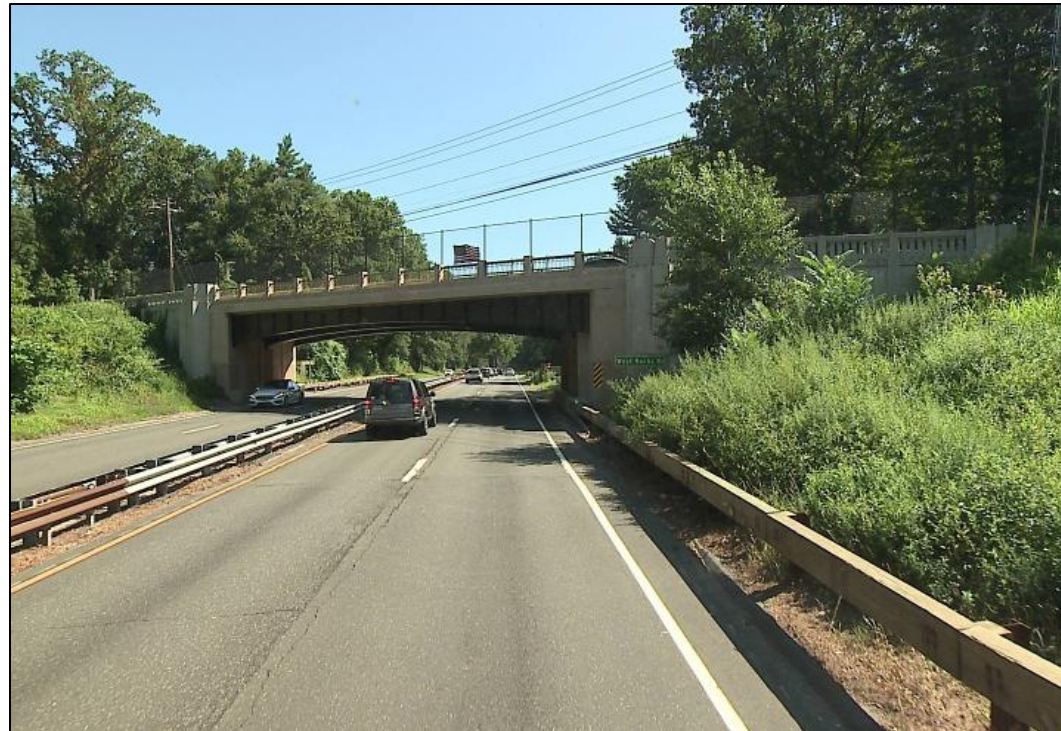
East side of bridge, facing west
