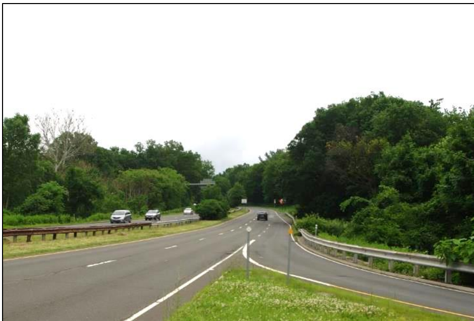
Parkway north of the Main Ave interchange, facing northeast
