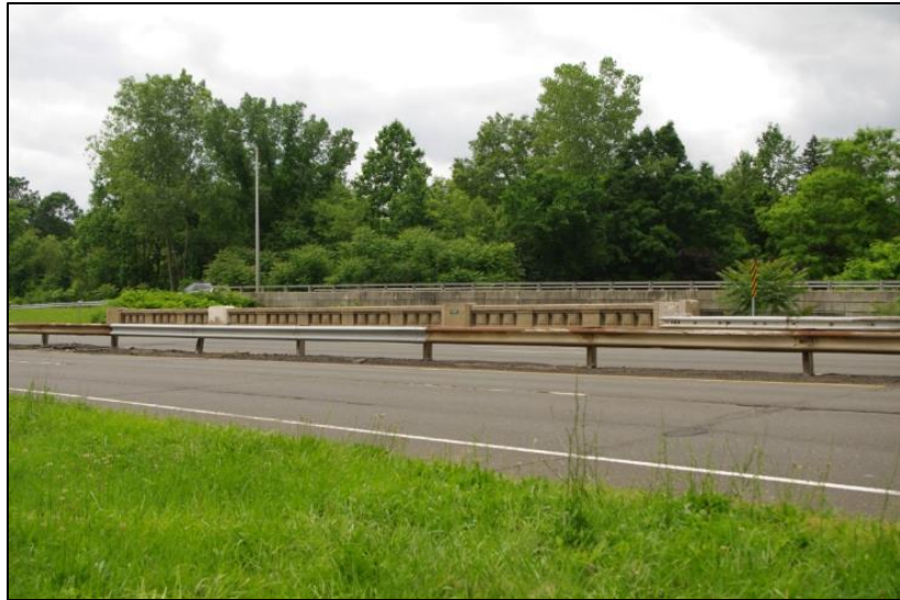
Perry Ave undergrade bridge, facing northwest. Northbound lane in foreground, guiderail, southbound lane, Perry Ave bridge parapet, and Route 7 Southbound-to-Parkway Southbound ramp
