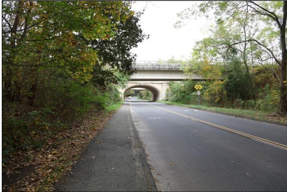
Existing view of south side as seen from Perry Ave, facing north
